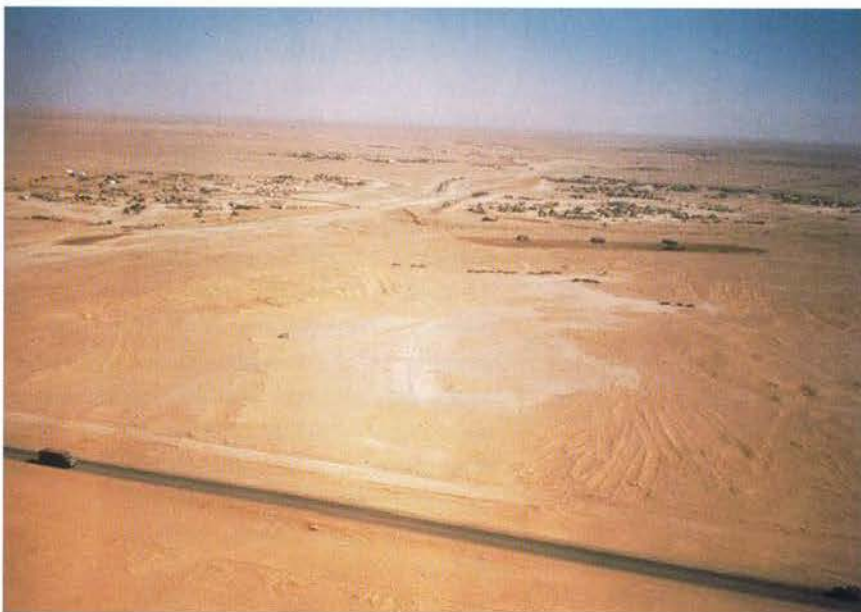
Tapline Road passing through logistical base CHARLIE
