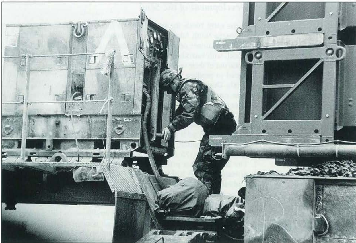
Starting one of two Patriot generators
