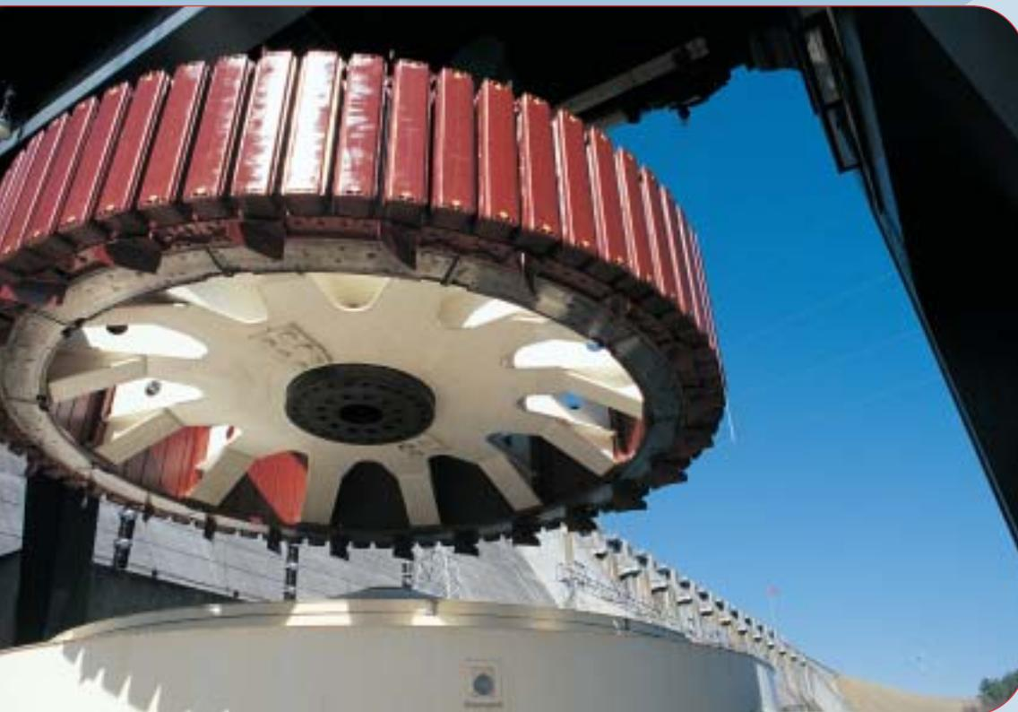
**(Left)** A 200-ton replacement rotor is moved into place at Georgia's Hartwell Power Plant, one of the Corps of Engineers' few external powerplants.
