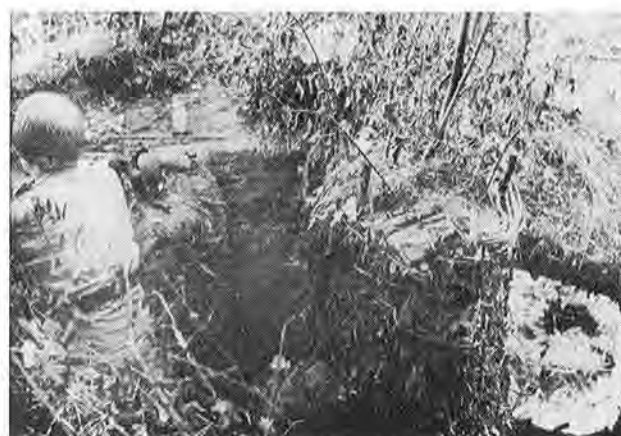
Typical German machine gun position. At the far right is the entrance to a shelter with a heavy log roof for protection against artillery fire.
