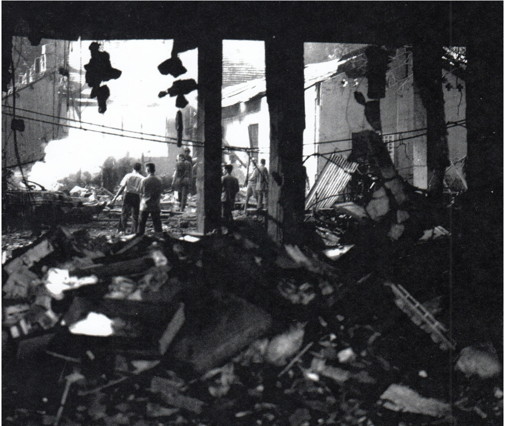
Bomb damage to the Brink Hotel
