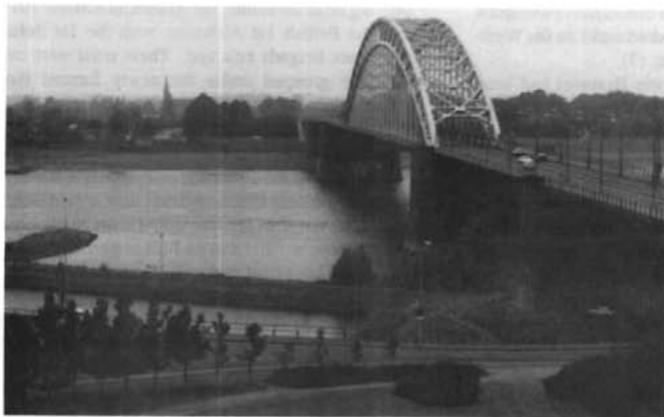
View of the Nijmegen bridge, looking north from the German command post.
