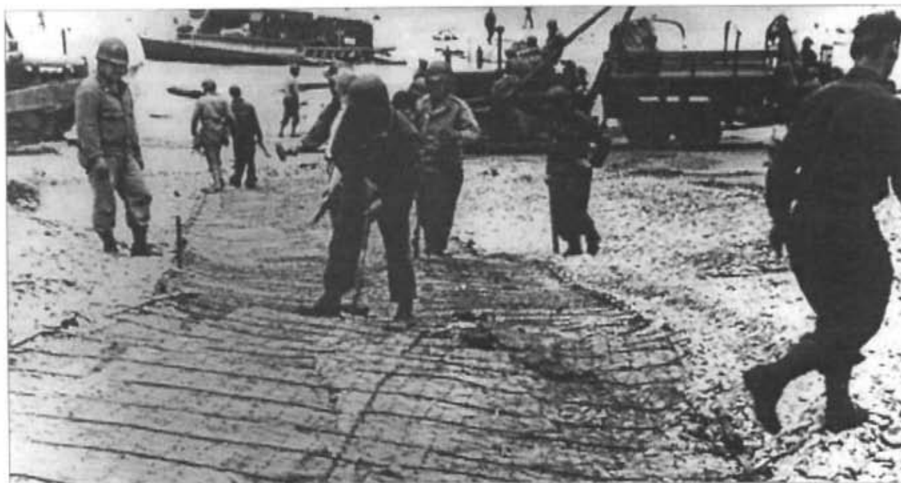
After landing on a beach in France, engineers lay out roads on the soft sands for the heavy vehicles and equipment yet to come ashore, 6 June 1944.
