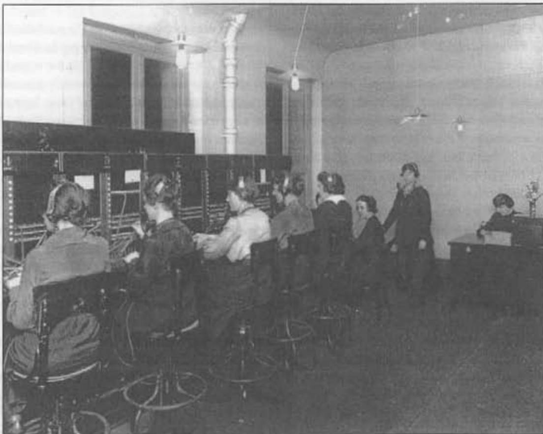
Signal Corps telephone switchboard operators at work in Bordeaux, France, with Nellie Snow at desk and Dorothy Sage standing (U.S. Army photo)
