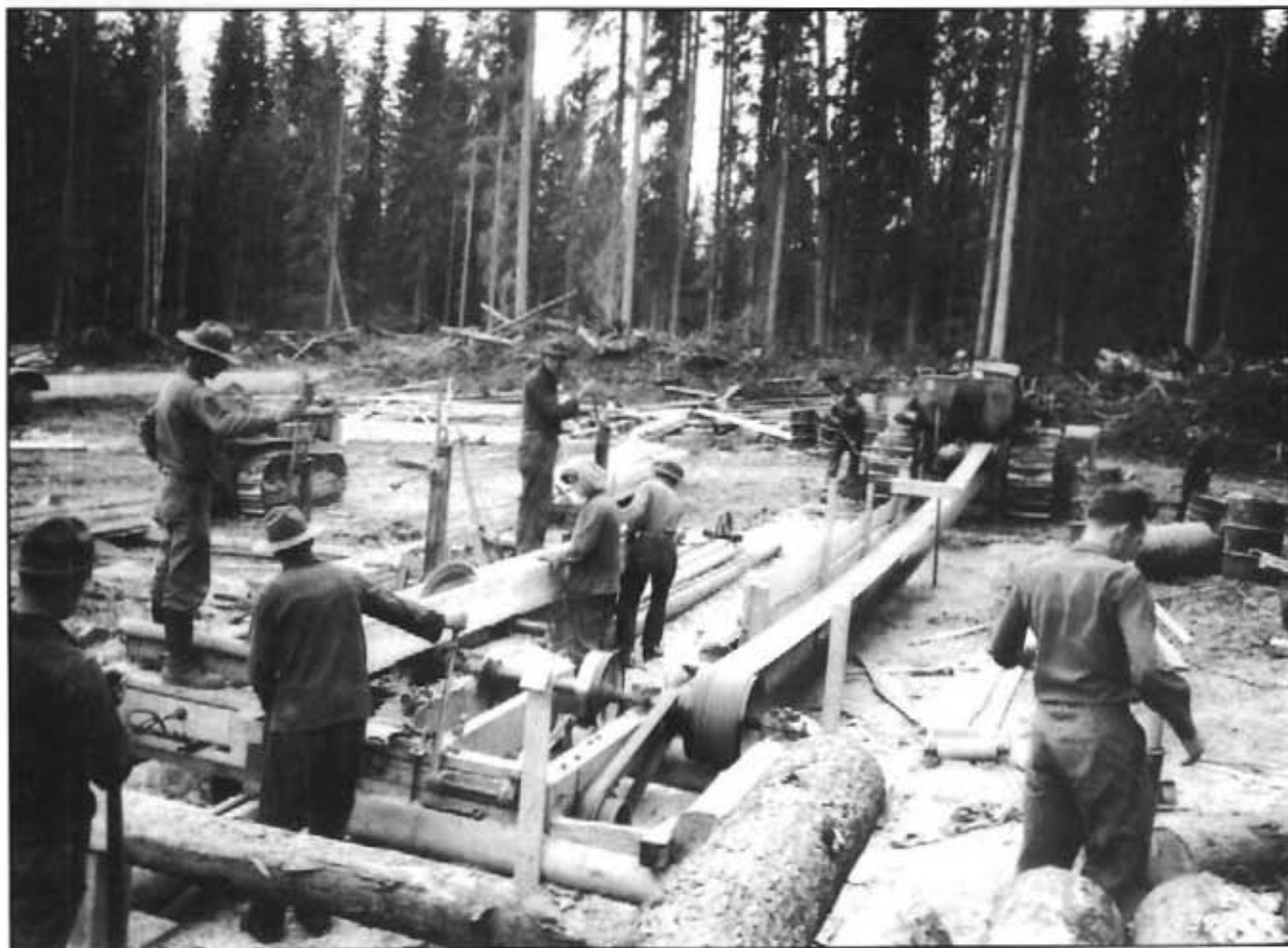
A D-8 Caterpillar tractor powers a makeshift sawmill along the Alcan Highway, 1942 (Signal Corps photo)
