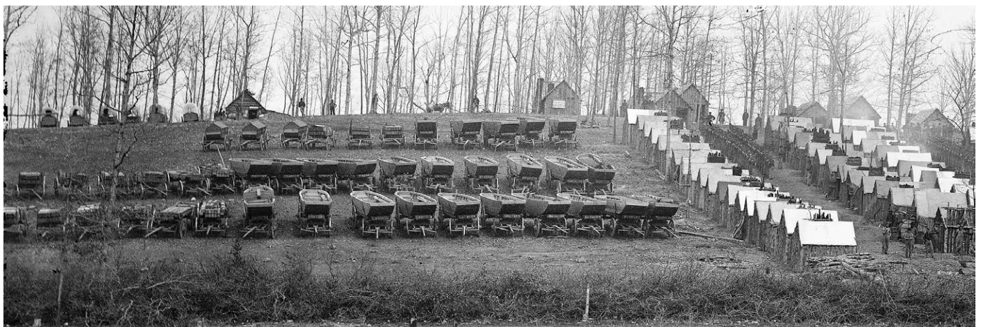
One of the wooden boat trains of the 50th New York Engineers at their camp near Rappahannock Station, Virginia, shortly before the beginning of the Overland Campaign Library of Congress
