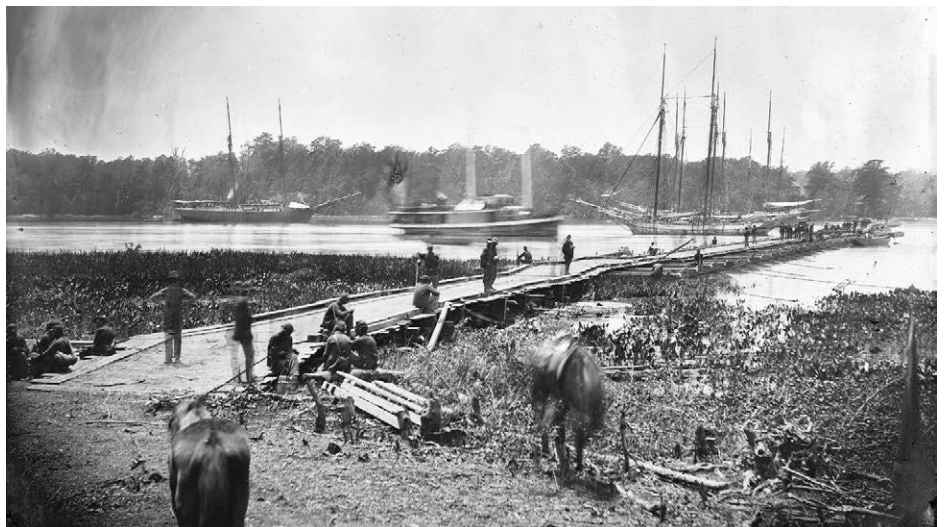
With boats in the water (center right) not attached to the main structure and soldiers clearly working atop the span, this photograph may show engineers constructing the pontoon crossing over the James River for Grant's move against Petersburg in June 1864.
