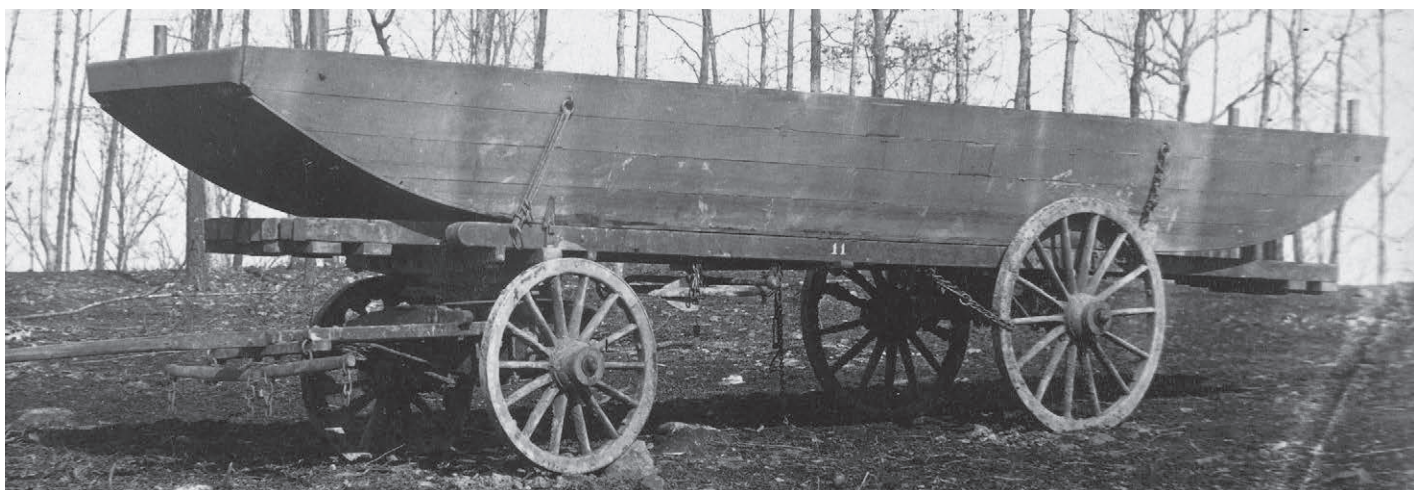
A wooden bateaux loaded on its transport wagon at the camp of the 50th New York Engineers near Rappahannock Station, Virginia, during the winter of 1863–1864. Library of Congress
