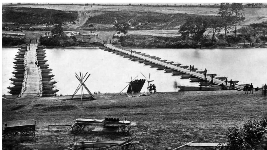
The construction of these bridges at the start of the Gettysburg Campaign exacted several casualties from the engineers, including Capt. Charles E. Cross, the commander of Company B, U.S. Engineer Battalion.
