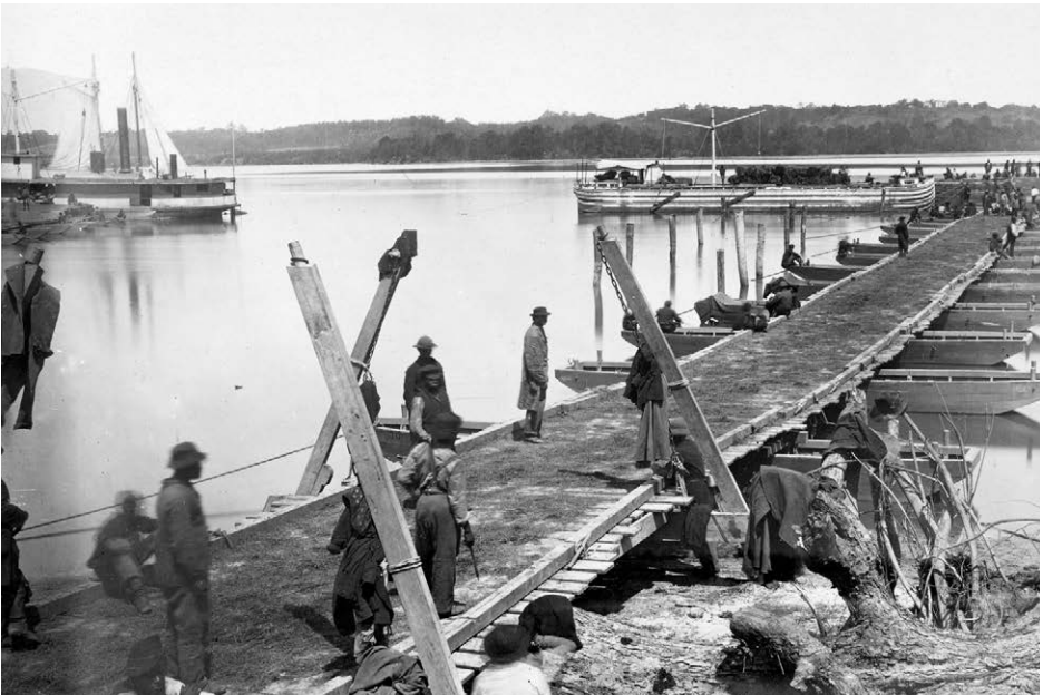
A pontoon bridge under construction at Belle Plain Landing, Virginia Library of Congress
