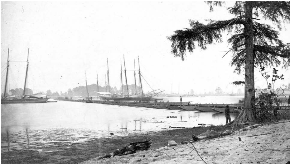
The completed bridge over the James in the late summer of 1864. This photograph also shows the heavy vessels used to stabilize it against the river's strong current and tidal changes.
