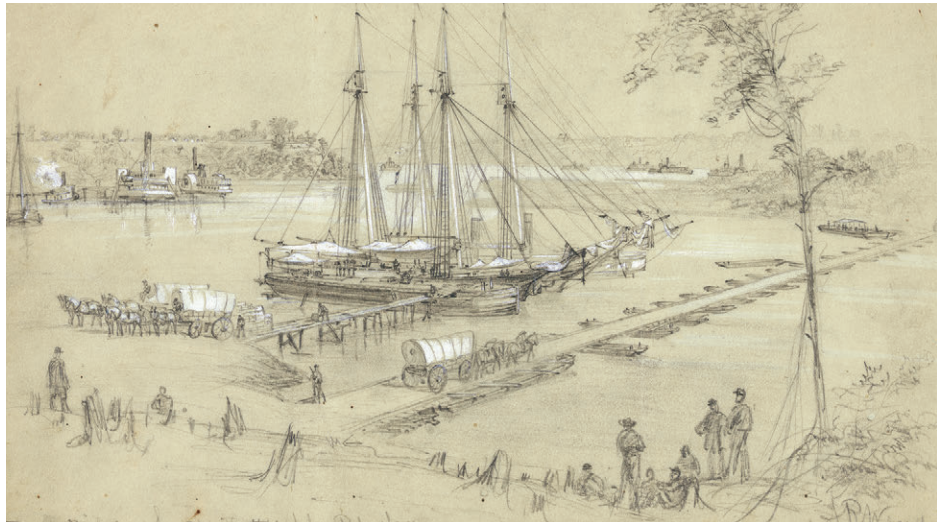
This July 1864 sketch by Alfred R. Waud shows the 1st New York Engineers' pontoon bridge at Point of Rocks on the Appomattox. They later disassembled the bridge and sent the boats downriver to aid in the effort to get the Army of the Potomac across the James River.
