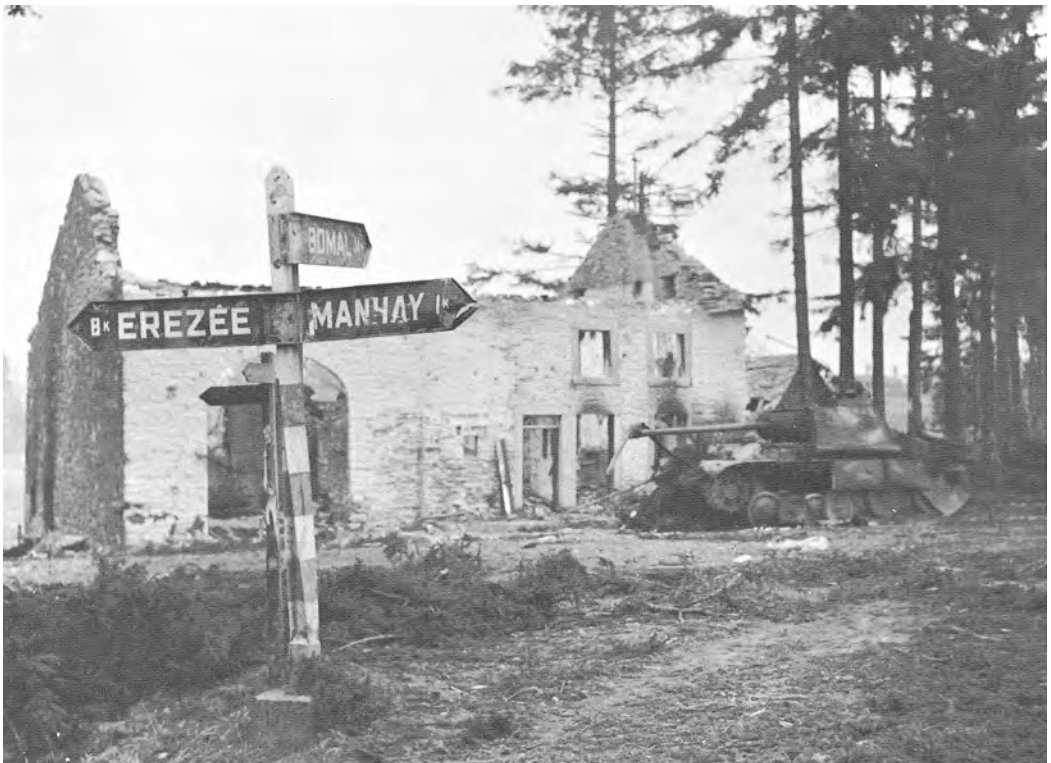
DESTRUCTION AT GRANDMÉNIL, including a damaged Panzerkampfwagen V (Panther).
