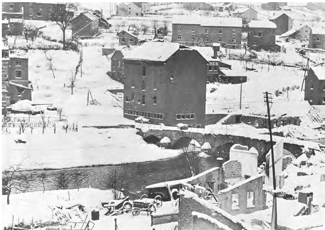
AMBLÈVE RIVER BRIDGE AT STAVELOT
