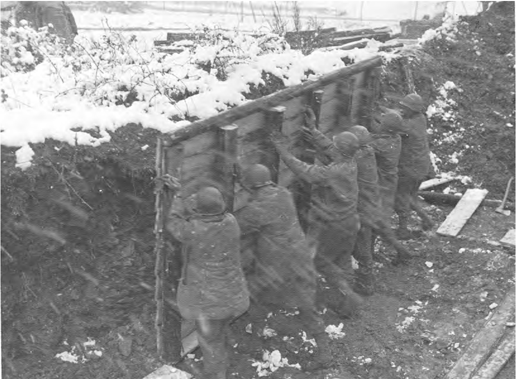
CONSTRUCTING A WINTERIZED SQUAD HUT NEAR THE FRONT LINES
