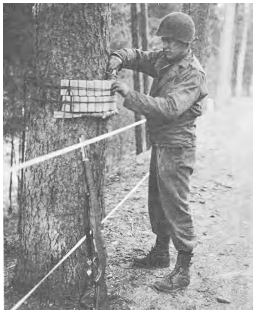
COMBAT ENGINEER SETTING A CHARGE. When the charge detonates, the tree will fall across the road to form part of a roadblock.
