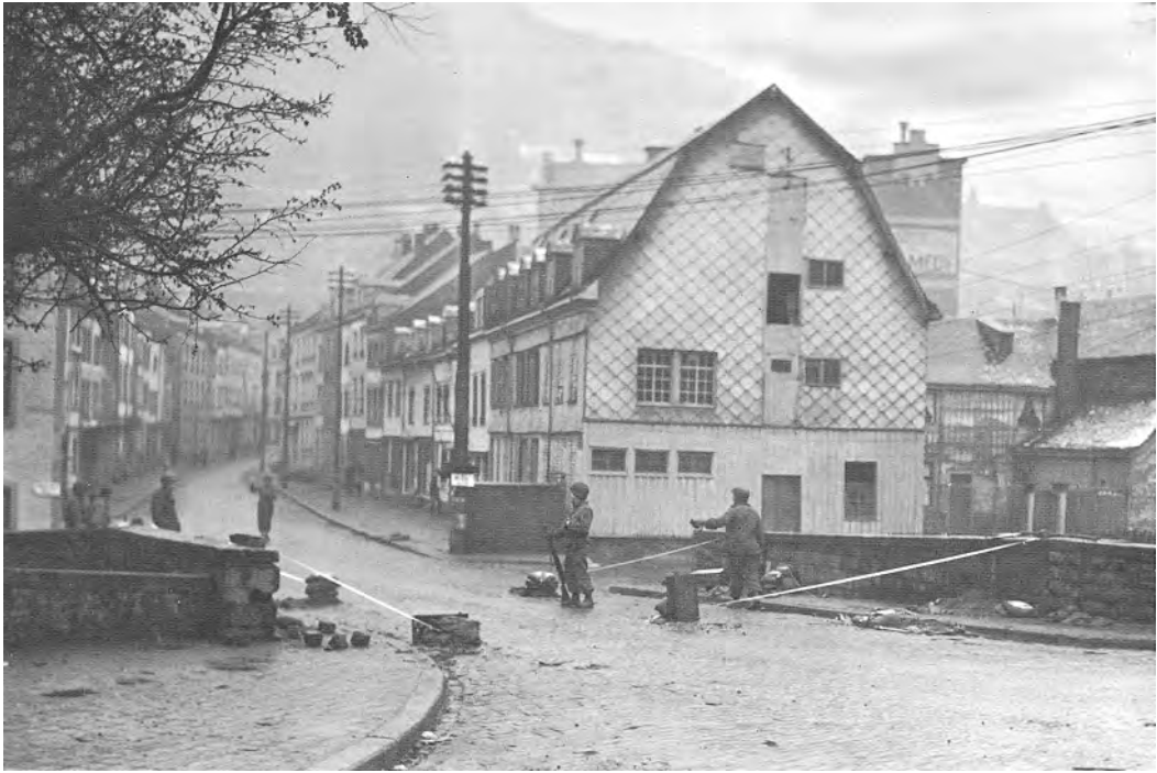
MINED BRIDGE IN MALMÉDY. Tapes mark safe passageway.
