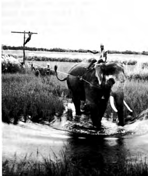
ELEPHANT DRAWS WIRE TAUT during pole line construction near Shampur, India. 31st Signal Construction Battalion.
