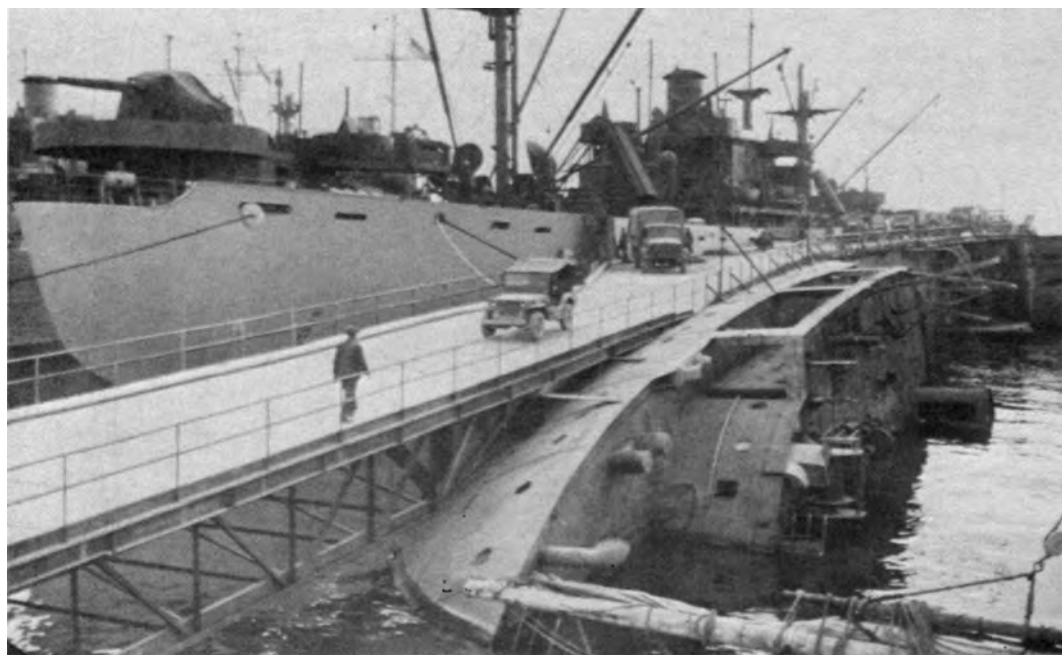
SUNKEN SHIPS in the harbor at Naples converted into piers for the berthing of Allied ships.
