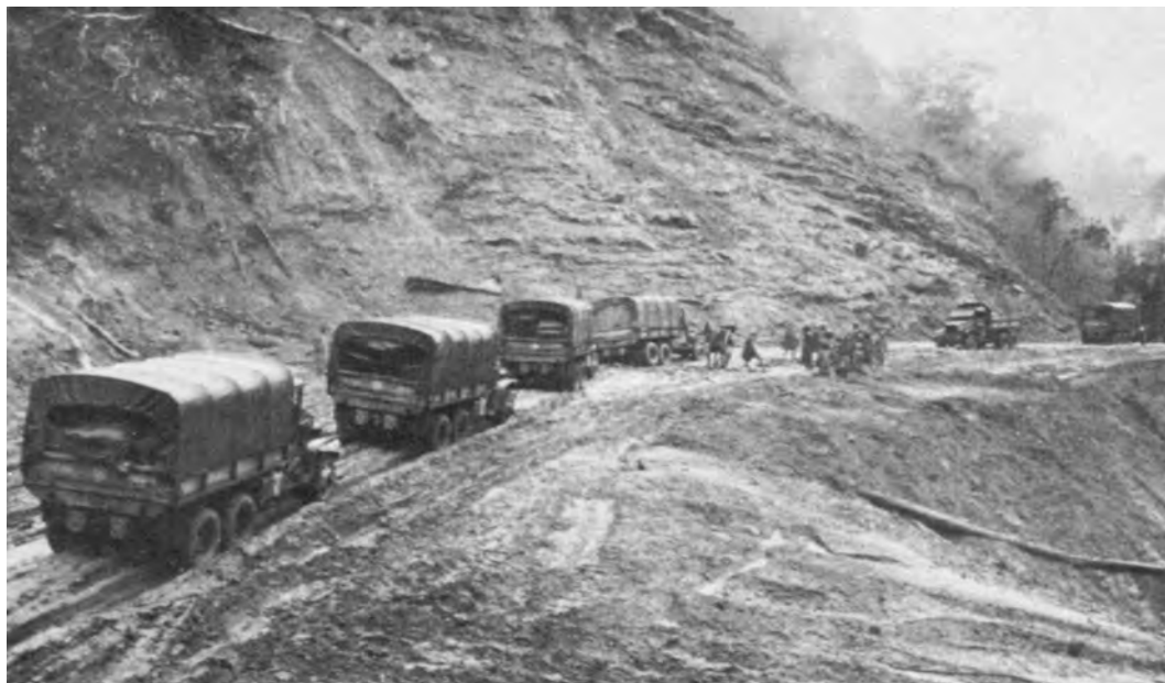
ROAD CONDITIONS IN BURMA AND IRAN ( above and below, respectively ). During the monsoon periods in Burma mud delayed deliveries. In Iran dust storms caused similar delays.
