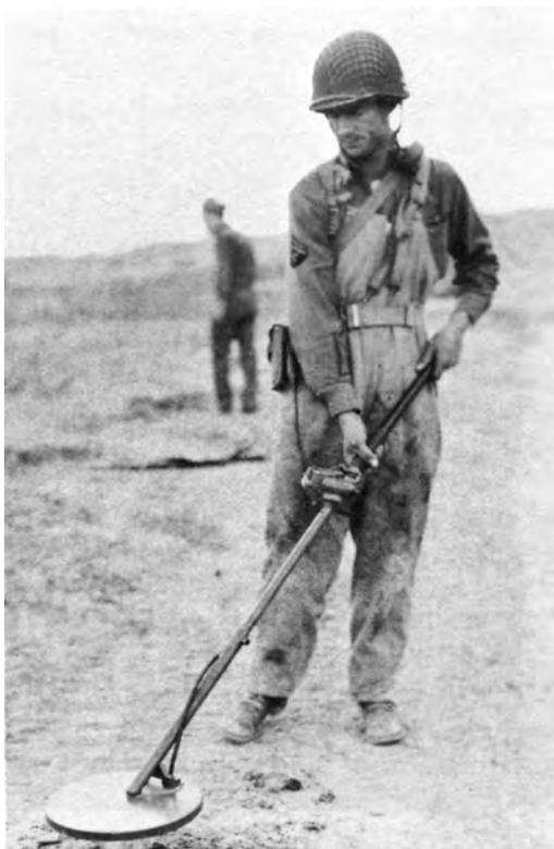
THE SCR-625 MINE DETECTOR *in action* on a Tunisian road.
