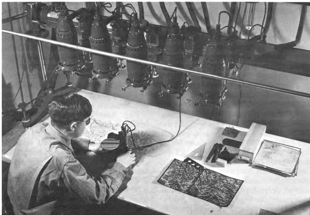
ENGINEER MAPMAKER USES A MULTIPLEX to establish accurate contours on invasion maps.
