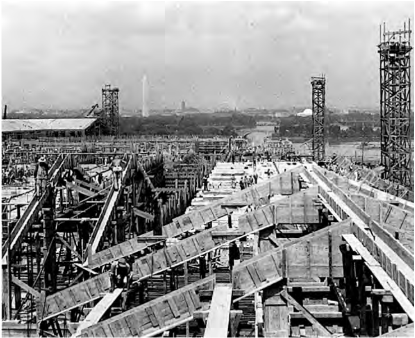
The Pentagon under construction. (DA photograph)
