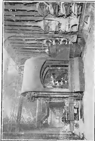
Retort house. Discharging machine drawing out the nearer half and pushing out the far half of the hot carbon.
