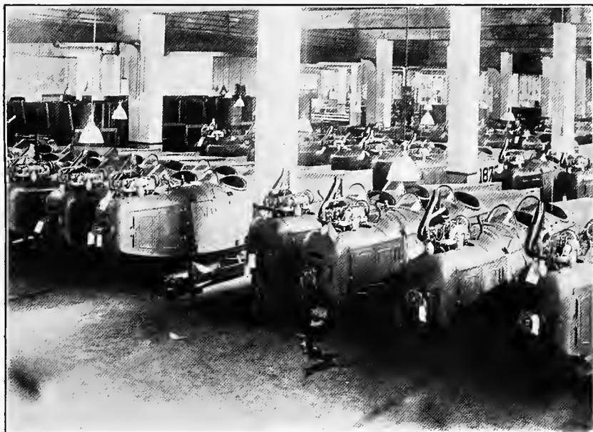
HALL-SCOTT ENGINES BEING INSTALLED IN AIRPLANE FUSELAGES.
