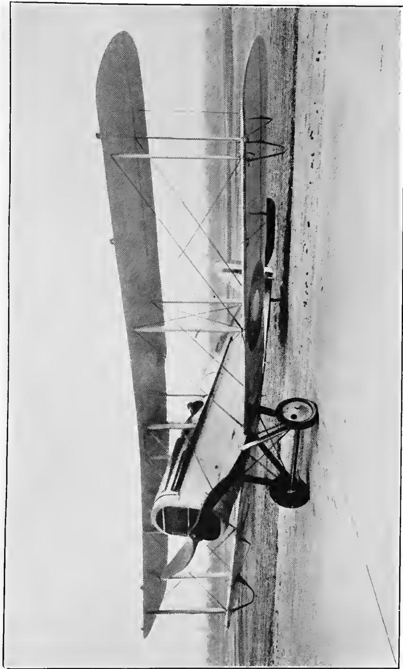
DE HAVILAND-4. USED FOR OBSERVATION, RECONNAISSANCE, COMBAT, DAY BOMBING, AND DEFENSIVE FIGHTING. Engines, Liberty 12, cylinder, 400-horsepower. Weight, empty, 2,391 pounds. Weight, full load, 3,582 pounds. Ground speed is 124.7 miles per hour. Speed at 10,000 feet, 117 miles per hour. Speed at 15,000 feet, 113 miles per hour. 10,000 feet is reached in 14 minutes with full load. Ceiling, 19,500 feet.
