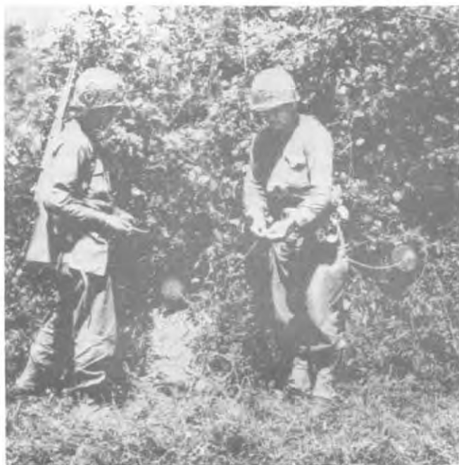
FIXING DEMOLITIONS to blow a gap through the hedgerow. Soldiers of the 121st Engineer Combat Battalion, who took part in the 29th Division drive, have loaded the holes made by tank prongs.
